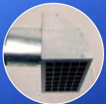
New air outlet duct
